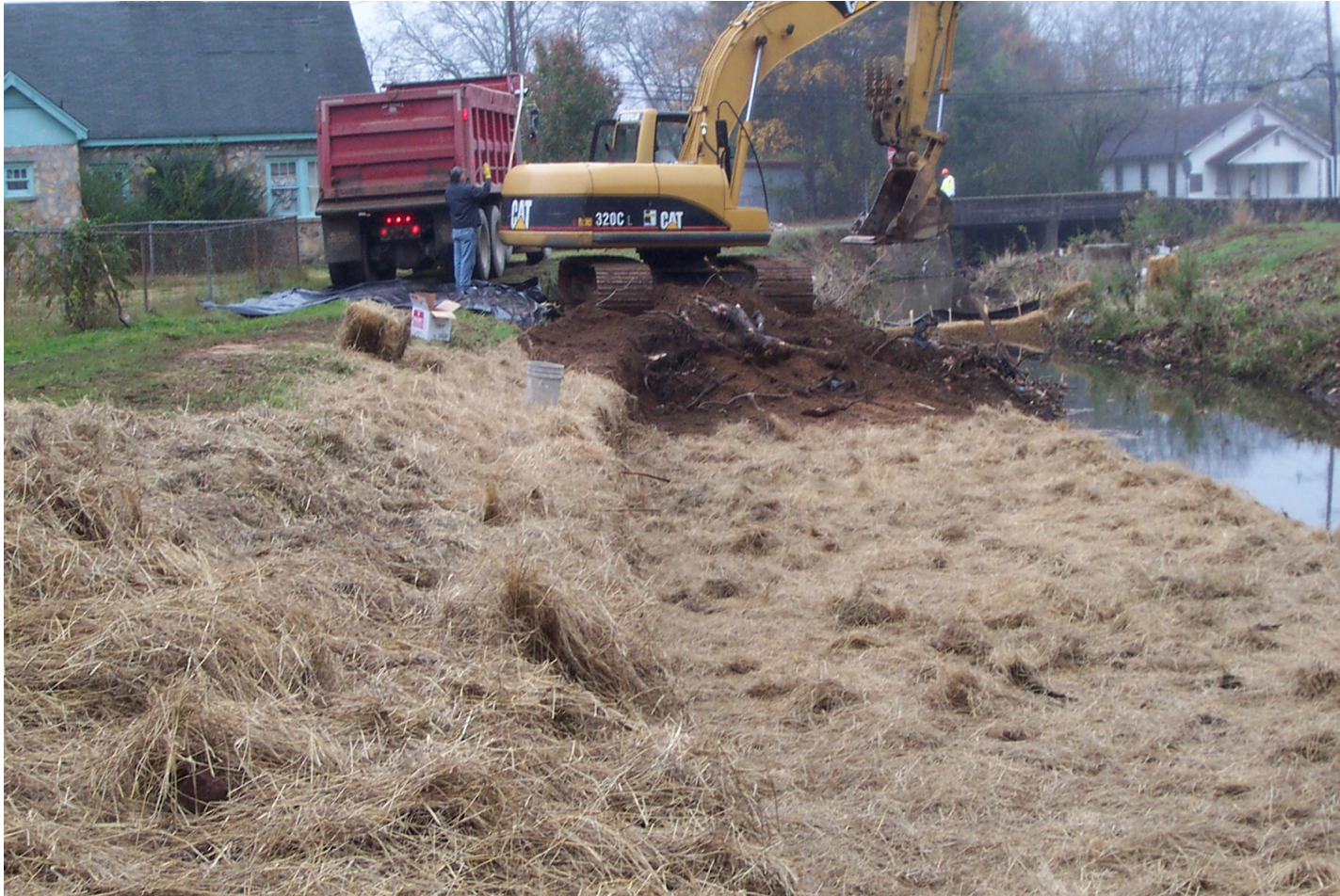
Removal from North Bank Side of Snow Creek - Facing East
