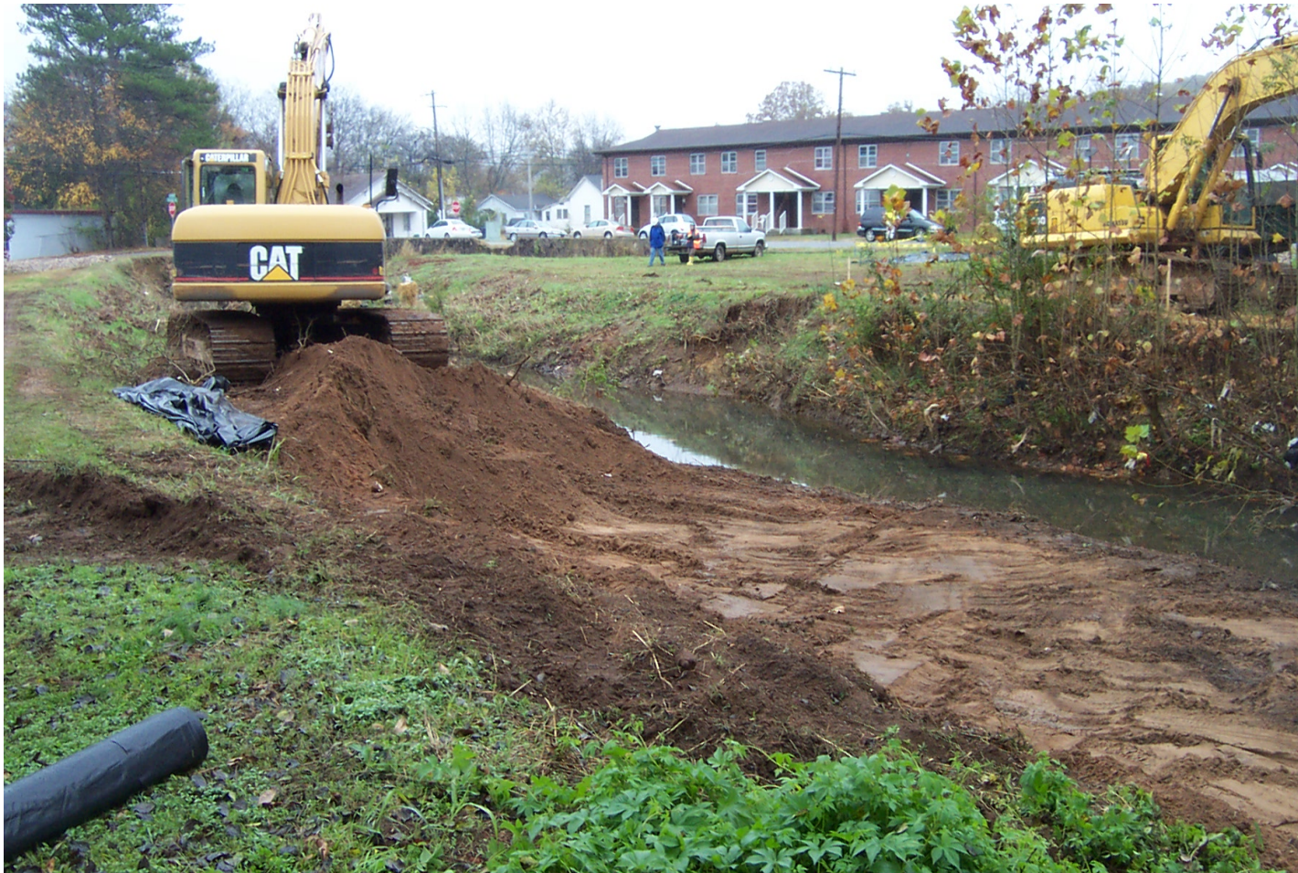
Removal from North Bank Side of Snow Creek - Facing South
